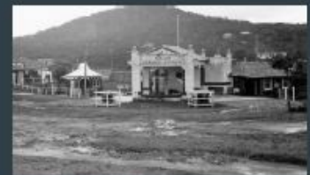
Service Station built circa 1927
