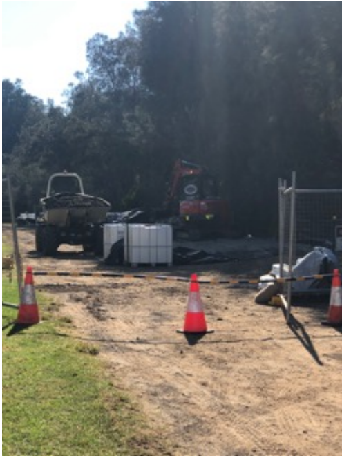
Careel Creek works Photo C Baker
